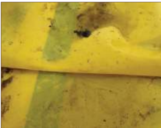
Figure A4.87 Tape joint with crease running through and air bubbles where gas membrane not in complete contact with tape. Rollers should have been used to produce a consistent seal (courtesy MEC Environmental Ltd)
