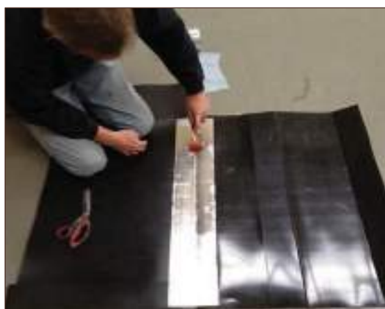
Figure A4.16 Example HDPE type gas membrane and steam roller used to ensure self-adhesive tape is correctly installed (courtesy A Proctor Group)
