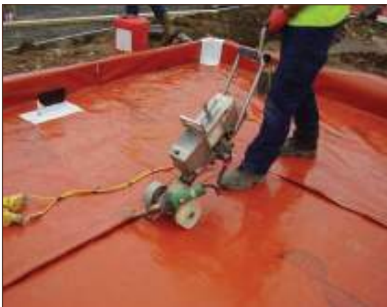
Figure A4.31 Extrusion welding (courtesy PAGEotechnical Ltd)
