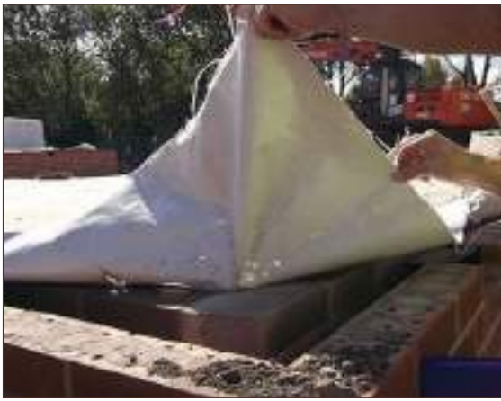
Figure A4.49 Lifted gas membrane at corner position. Light penetrating through confirms damage to aluminium internal core layer (courtesy NHBC)
