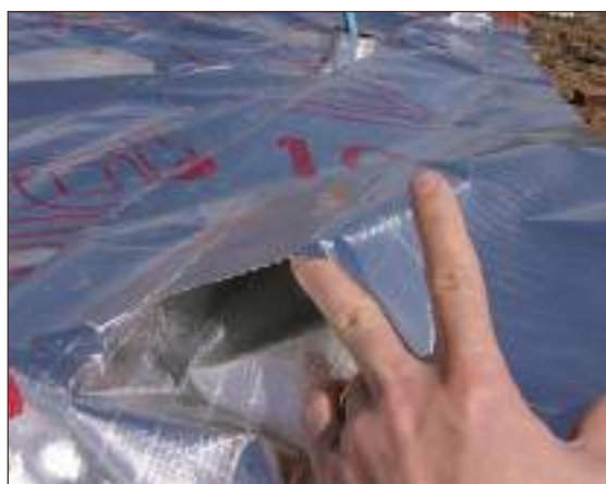
Figure A4.78 Gap in jointing over wall cavity big enough to insert fist (courtesy Smith Grant)
