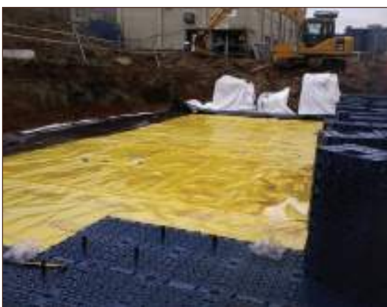
Figure A4.17 Gas membrane installed in attenuation tank (courtesy Industrial Textiles & Plastics Ltd)
