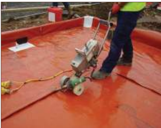
Figure A4.31 Extrusion welding (courtesy PAGeotechnical Ltd)
