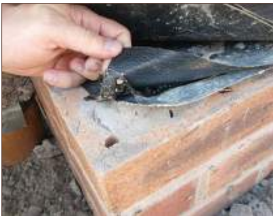
Figure A4.13 Gas proof DPC adhered on top of gas membrane using butyl strips across cavity space (courtesy NHBC)
