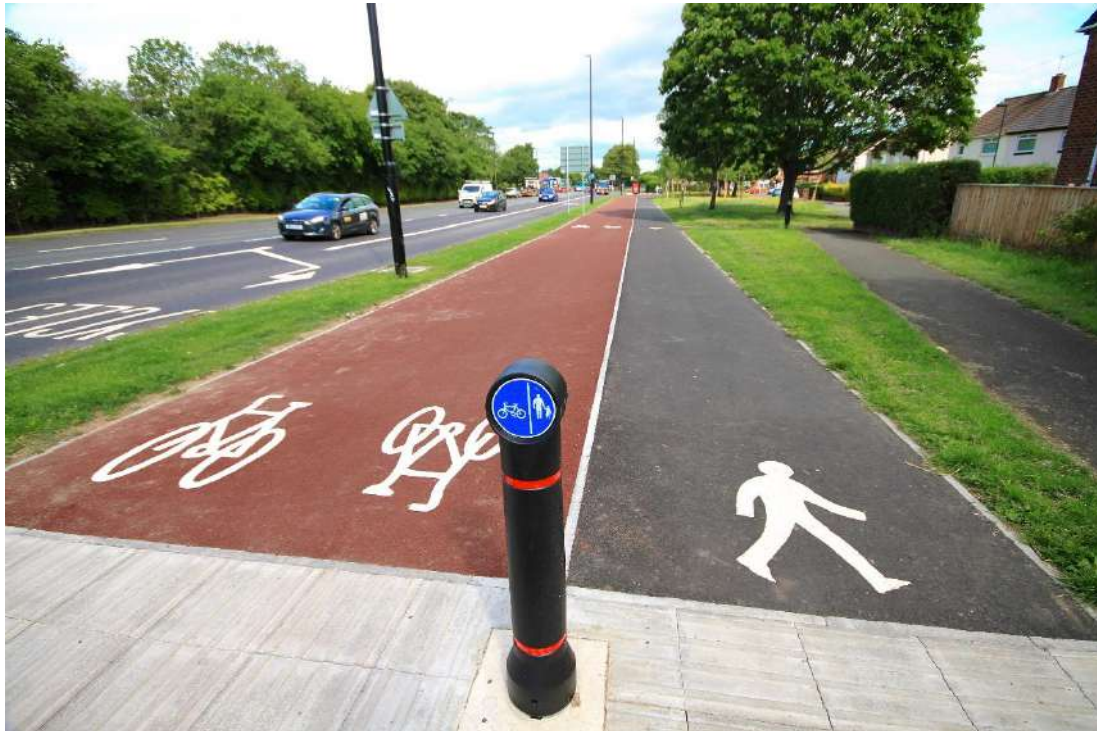
Image 1 – Two-way segregated cycle track in Longbenton, North Tyneside
